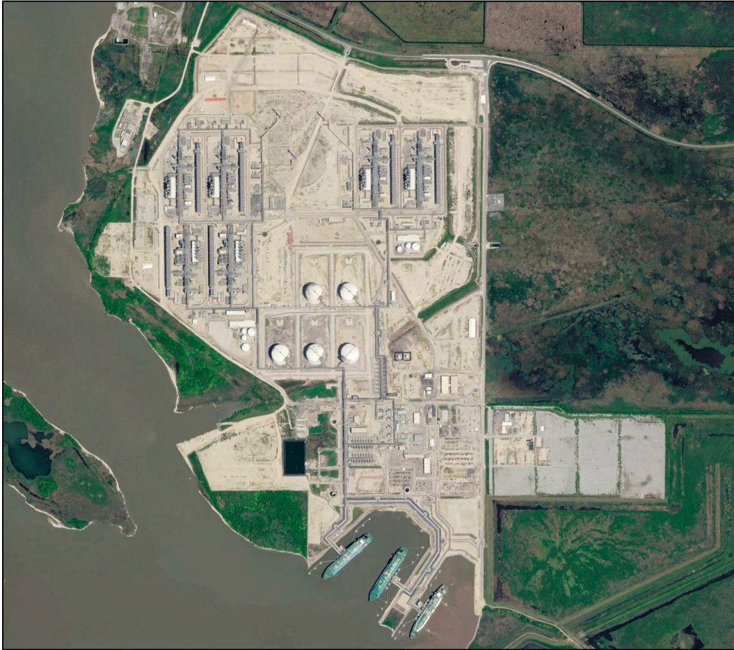
Figure 3: Aerial view (dated 4/7/2025) of the Sabine Pass LNG export facility
